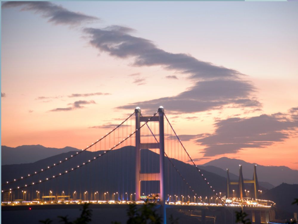
Tsing Ma Bridge
